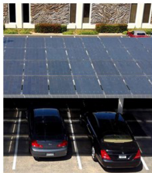
Example of installation in Sunnyvale, CA 1
