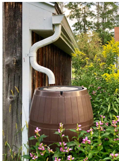
Example of a potential rainwater harvesting system.
