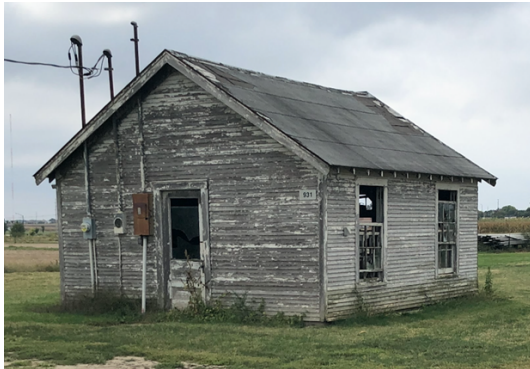
Building 931 (first building to have CornCrete installed)
