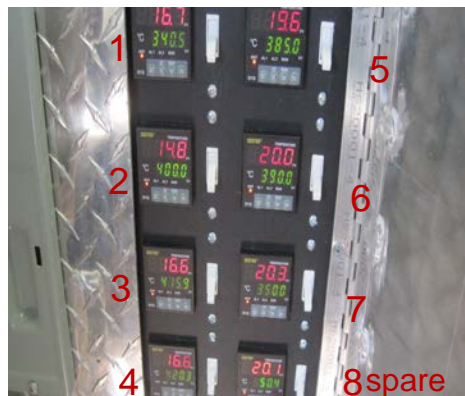
Temperature controllers and the zones they control
