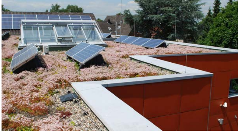
Figure 1: Rooftop created by Green Roof Technology that combines solar panels with a green roof (Green Roof Technology 2015).
