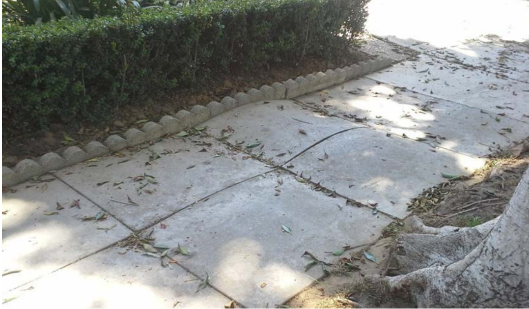
Figure 2: Terrewalk sidewalk panels shown expanding around tree roots (Mendiola 2017)
