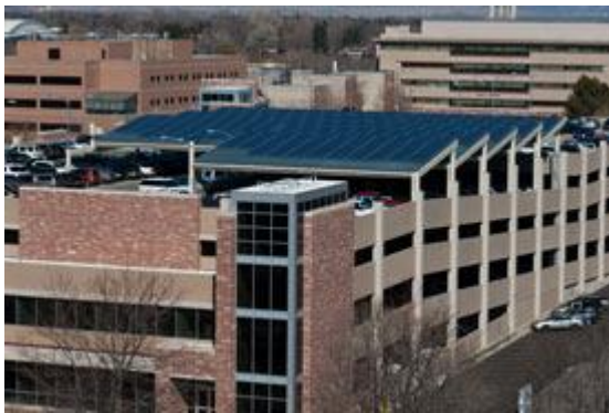
Fig. 1. Parking structure at Colorado State University
