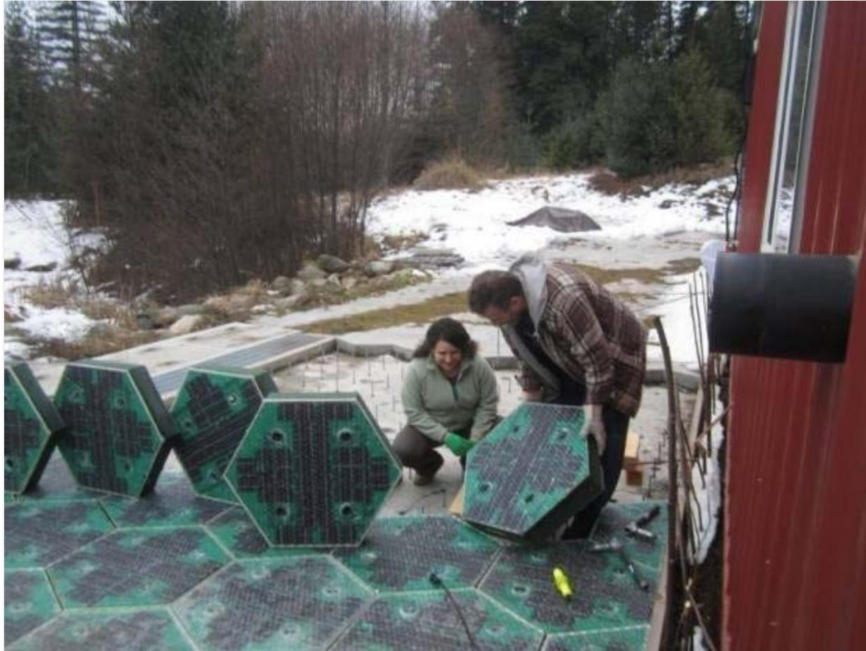
Figure 1. Solar RoadWays panel installation(Solar RoadWays, 2014)
