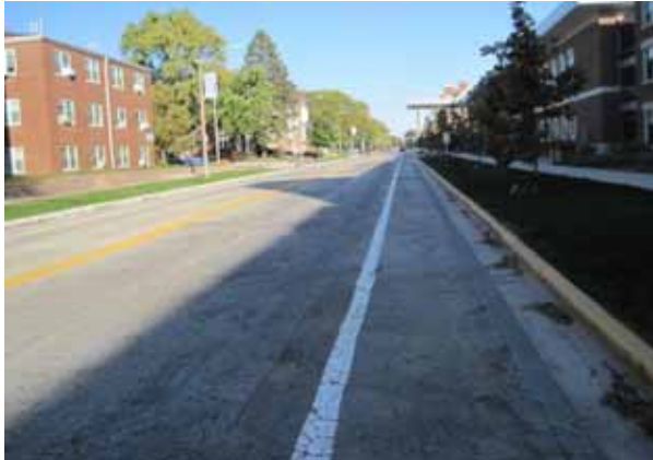
Existing Bicycle Lane on Gregory Drive near Ikenberry Commons (#240) Photo by Holly Nelson
