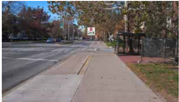
Green Street at Mathews Avenue, where existing side path goes through a bus stop (#150) Photo by Geoff Merritt
