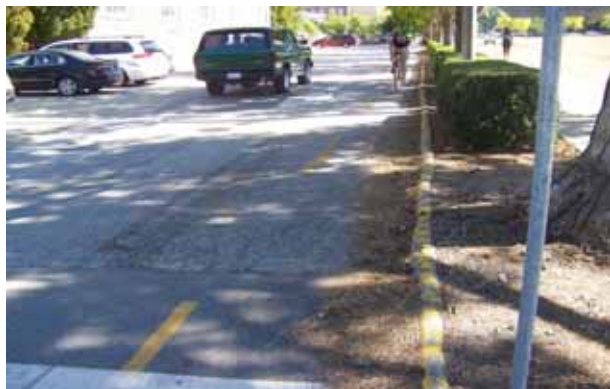
Existing Dedicated Bike Path runs through the Huff Hall parking lot, with little to no separation from cars (#770) Photo by F&S
