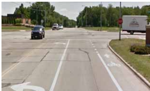
Existing Shared Use Path along Race Street (#400) Photo by F&S
