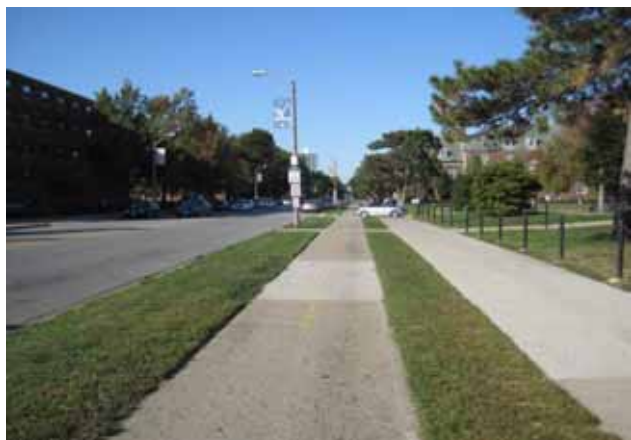
Existing Dedicated Bicycle Side Path along Fourth Street (#260). Photo by Holly Nelson
