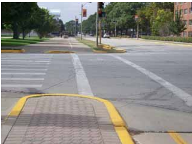
Segment #355 as seen from #357 Photo by F&S
