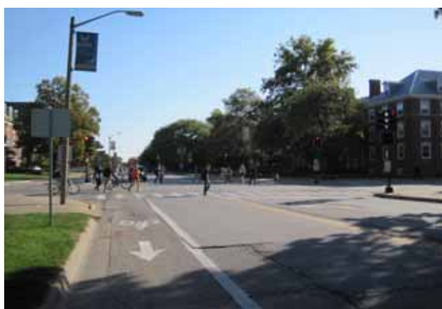
Existing Bicycle Lane along Fourth Street north of Gregory Drive (#260). Photo by Holly Nelson
