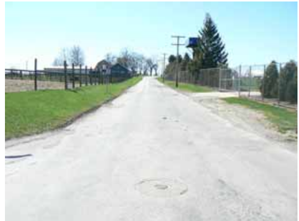
St. Mary's Road (#430) Photo by CCRPC
