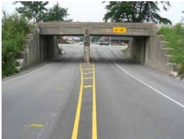
St. Mary's Road passes under the railroad and intersects with Neil Street (#410). Photo by CCRPC
