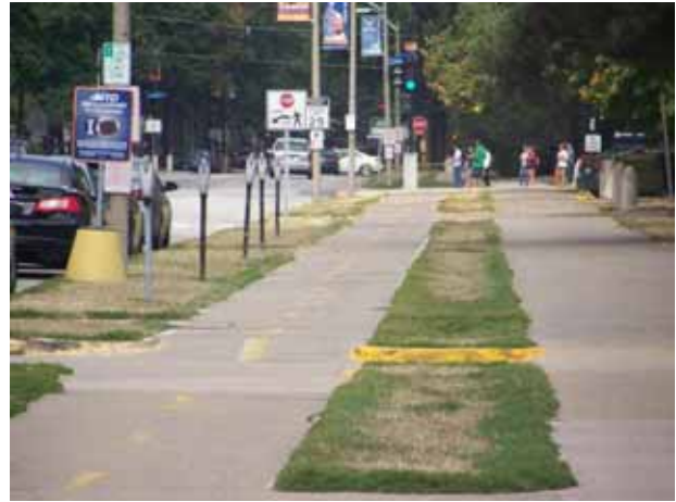
Existing Dedicated Bicycle Path (#355) Photo by F&S
