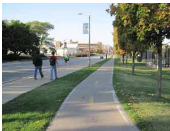
Existing Dedicated Bicycle Side Path along Dorner Drive (#290) Photo by Holly Nelson
