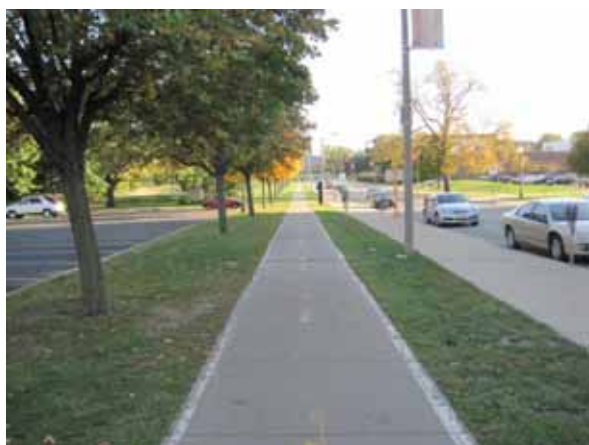
Existing Dedicated Bicycle Side Path along Dorner Drive (#290) Photo by Holly Nelson
