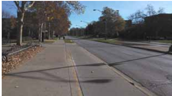
Green Street east of Goodwin Avenue, where existing side path ends mid-block (#150) Photo by Geoff Merritt
