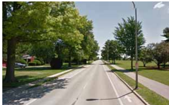
Existing Shared Use Path along Race Street (#400) Photo by F&S
