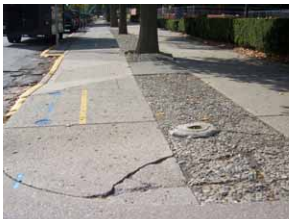
Existing Dedicated Bike Path along Mathews Avenue (#70) Photo by F&S
