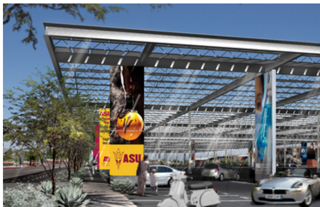
Figure 5. ASU Solar Canopy
