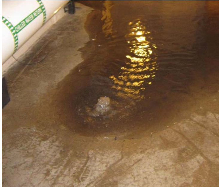
Figure 3-3 Opening in Tunnel Immediately South of Noyes Hall
