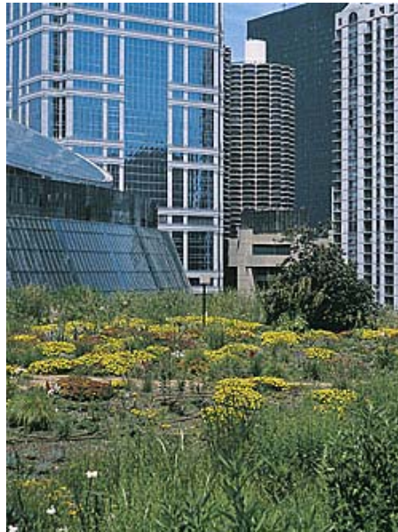
Figure 4-17 Green Roof – Chicago City Hall
