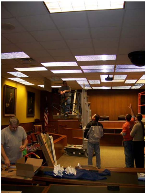
Figure 1: Law Building Retrofit in Progress
