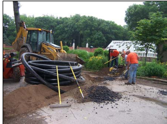
Water line installation
