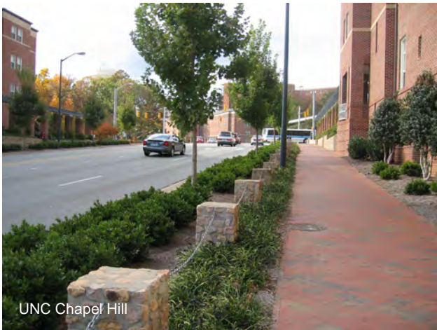
Pedestrian channelization treatment at UNC Chapel Hill. Combines landscaping with attractive stone bollards to direct pedestrians to the signalized intersection.
