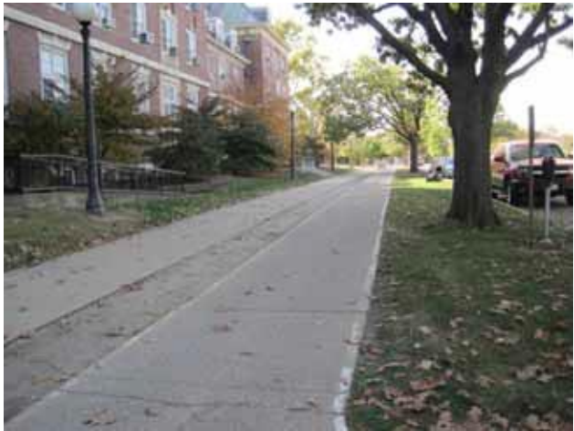
Existing Dedicated Bicycle Side Path along Peabody Drive (#357) Photo by F&S
