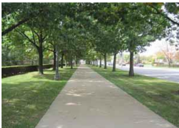
Existing Shared Use Side Path along University Avenue (#10) Photo by Holly Nelson
