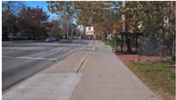
Green Street at Mathews Avenue, where existing side path goes through a bus stop (#150) Photo by Geoff Merritt
