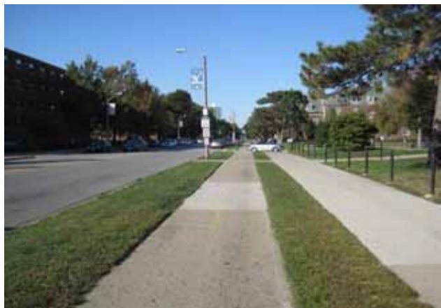
Existing Dedicated Bicycle Side Path along Fourth Street (#260). Photo by Holly Nelson
