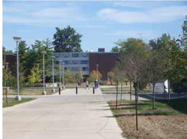
Existing Shared Use Path Lorado Taft Path in Ikenberry Commons (#780) Photo by Andy Kopp
