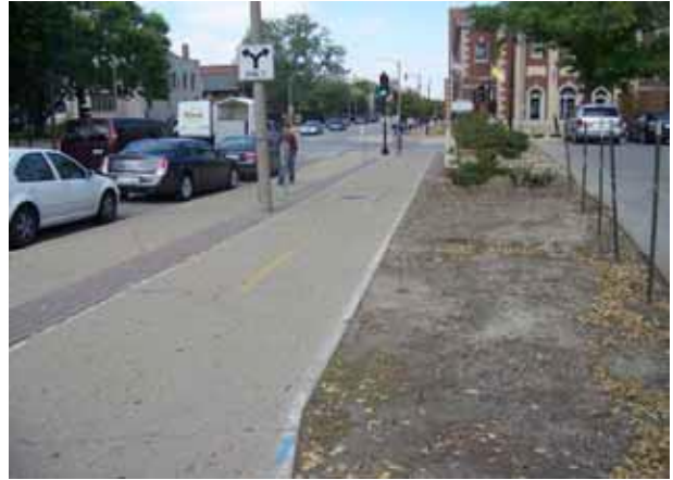
Existing dedicated bicycle path (#270) Photo by F&S
