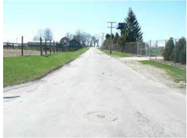
St. Mary's Road (#430) Photo by CCRPC
