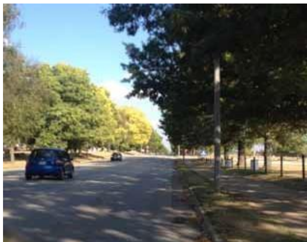
Existing Shared Use Path along Florida Avenue (#390)
