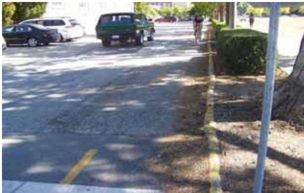
Existing Dedicated Bike Path runs through the Huff Hall parking lot, with little to no separation from cars (#770) Photo by F&S
