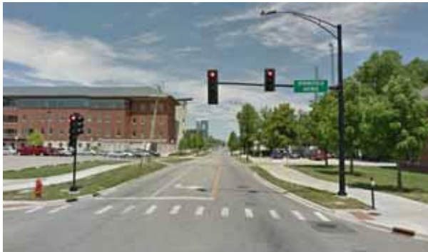
Existing Shared Use Path along Goodwin Avenue (#20) Photo by F&S
