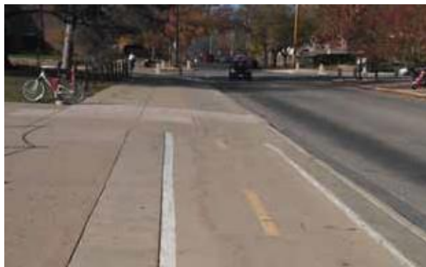
End of side path along Armory Avenue (#100) Photo by Geoff Merritt
