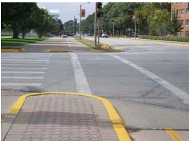
Segment #355 as seen from #357 Photo by F&S
