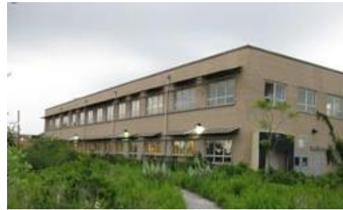
Figure 10. Chicago Center for Green Technology Solar Awnings
